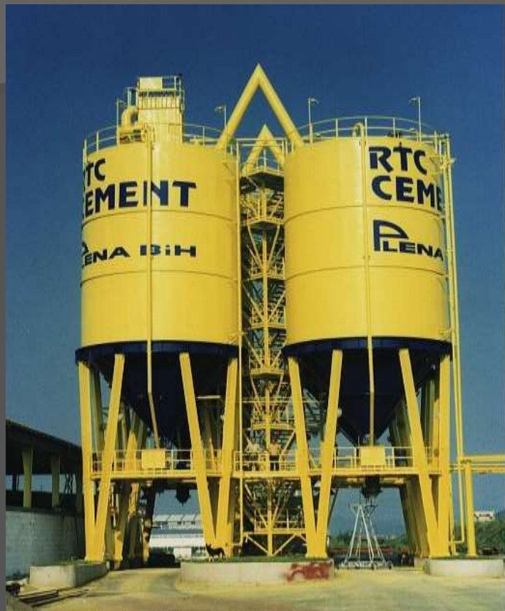
Cement silos in Bosnia & Herzegovina capacity 2000 t.
